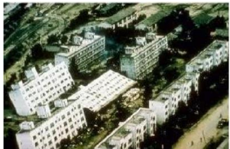
Examples of liquefaction consequences (NASEM, 2016)
