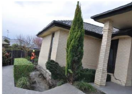
Examples of liquefaction consequences (NASEM, 2016)
