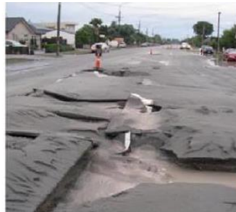
Examples of liquefaction consequences (NASEM, 2016)
